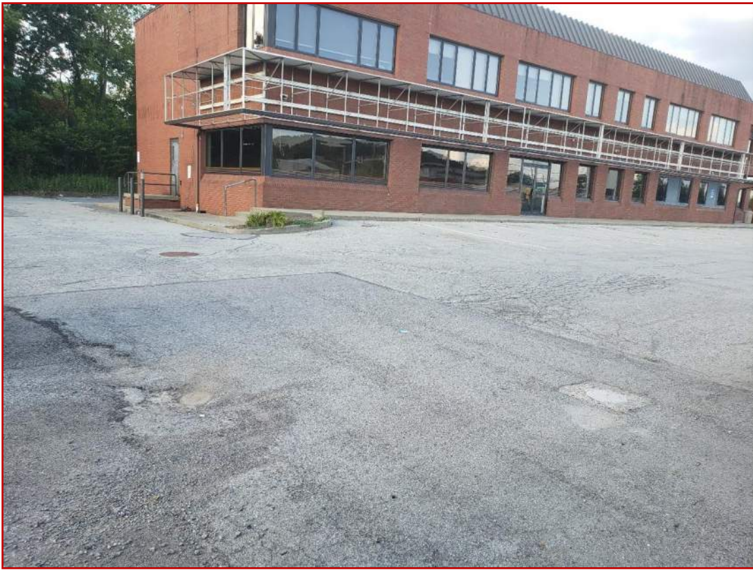
Photo 1: View of former 7-11 Gas Station near Franklin Road– Facing Northeast (8.11.20)
