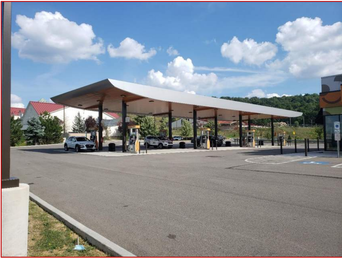
Photo 9: American Natural fueling dispensers – Facing Southeast (8.11.20)
