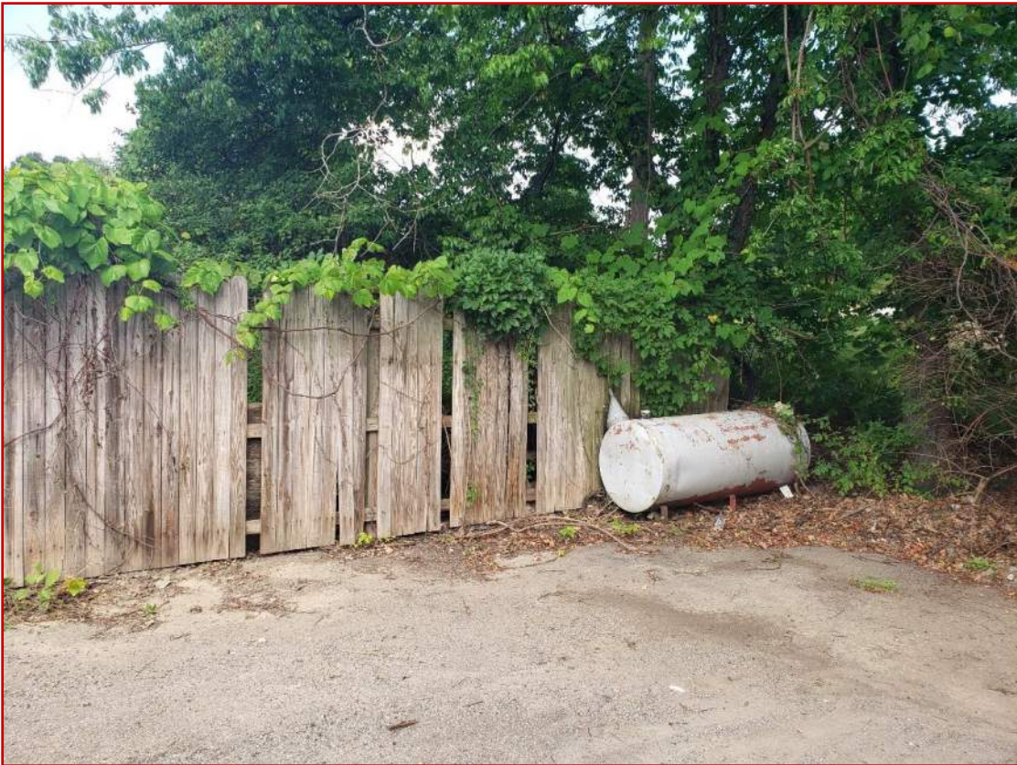
Photo 4 : Above ground tank located on former Grabenstein Texaco property – Facing Northeast (8.11.20)
